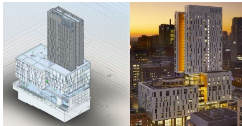
PHOTO: EXAMPLE OF DIGITAL TWIN MODEL (LEFT) OF EXISTING BUILDING (RIGHT) FROM BOOTCAMP WORKSHOP
